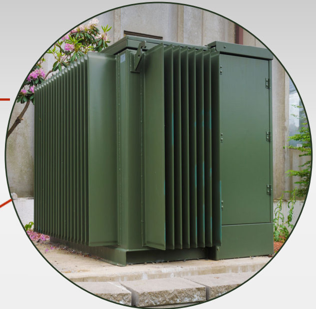
Step Down Transformer
